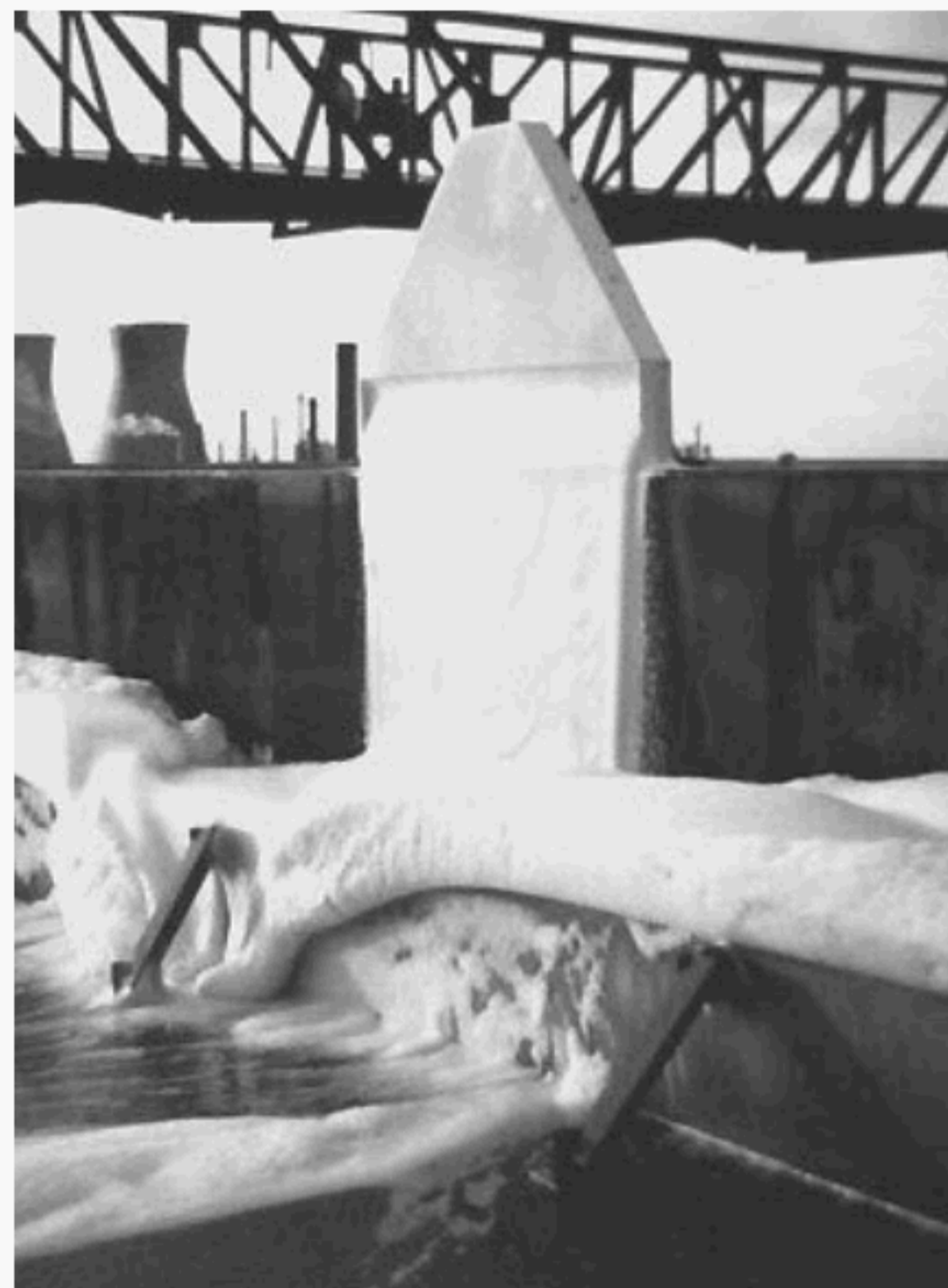
Figure 12—Foam for Seals Flowing into Foam Dam from Permanently Installed Foam Chamber
