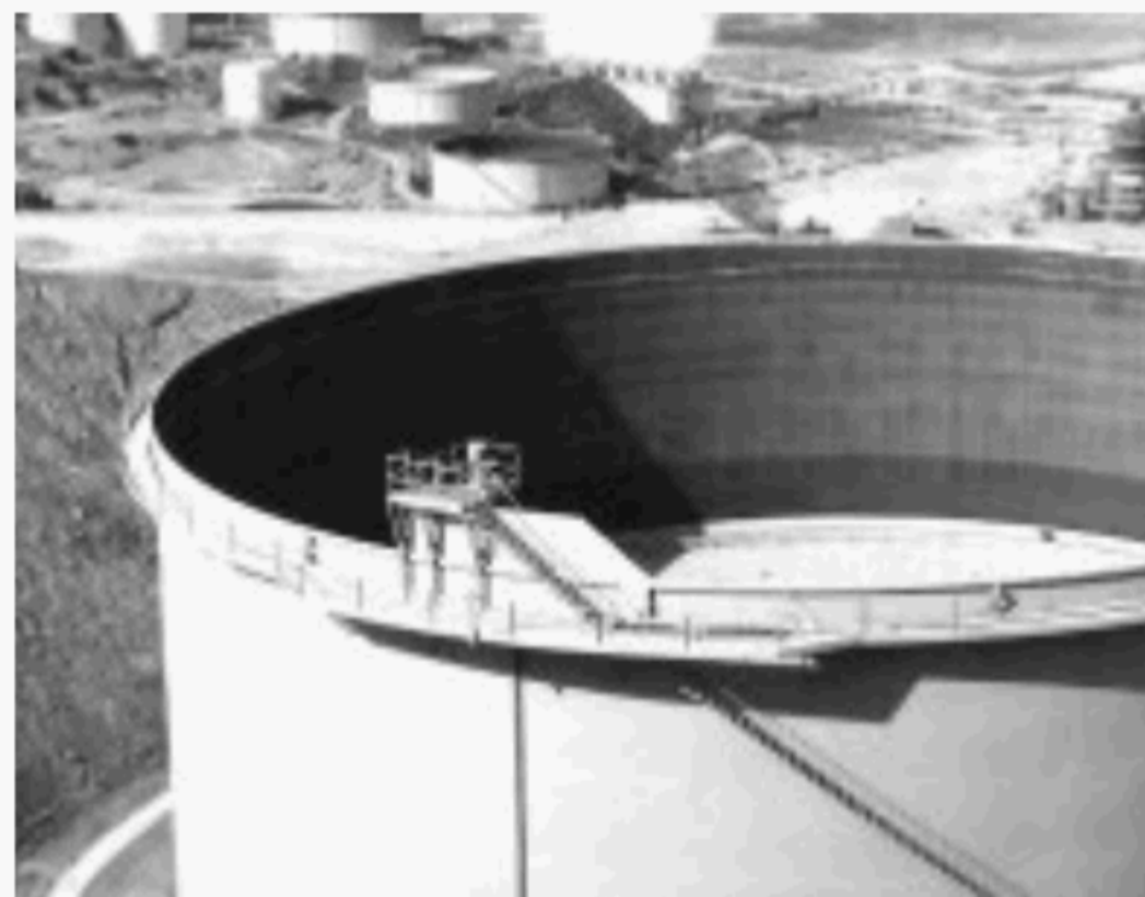
Figure E-6a—Open Top (External) Floating Roof Tank
